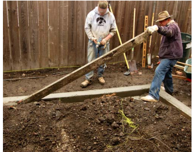
Pulling the forms
