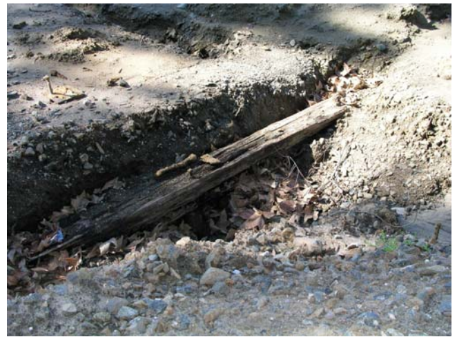
Historic trestle bent just discovered at CSRM
