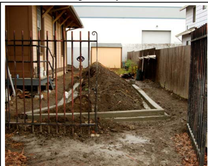
First Stage Foundation
