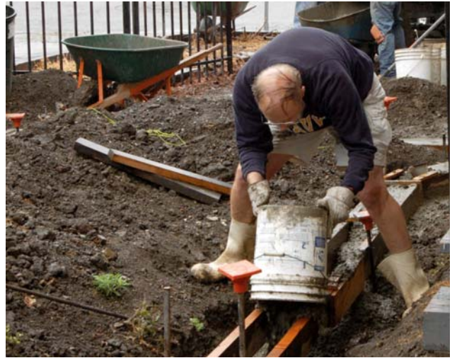
Joe Barker placing concrete one bucket at a time.
