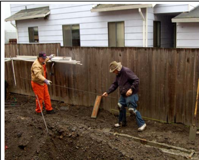
Pat LaTorres & Bill Alexander placing re-bar.
