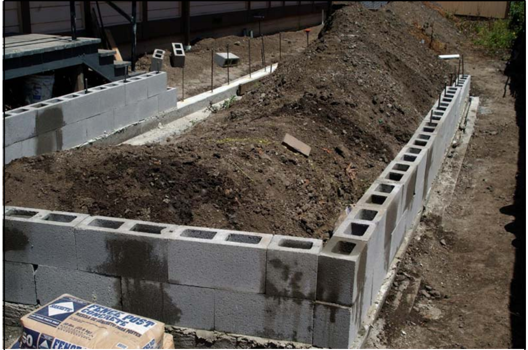
Finished children's wall, ready for soil.
