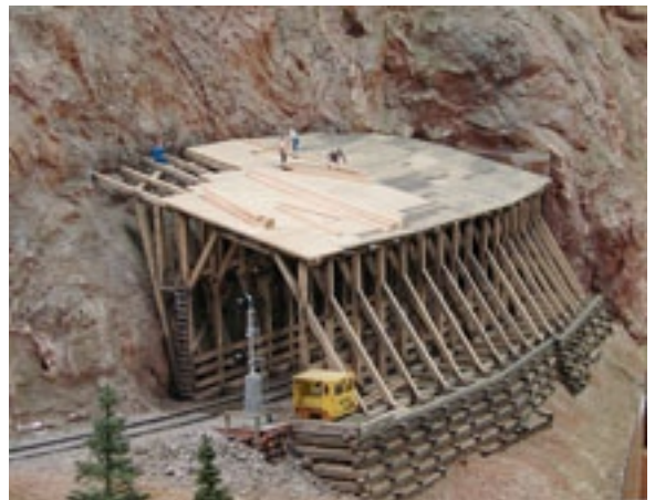
Snow Shed Under Construction
