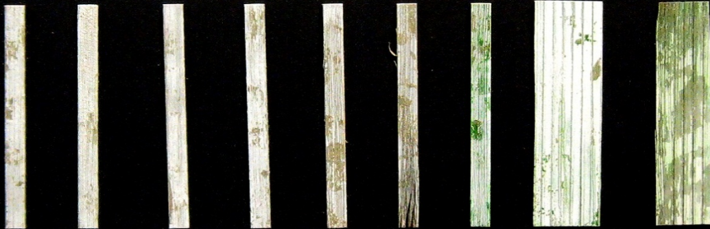
Peeling Paint Examples 1-5 Rotting bottom Peeling paint on Peeling paint 1 - 3
