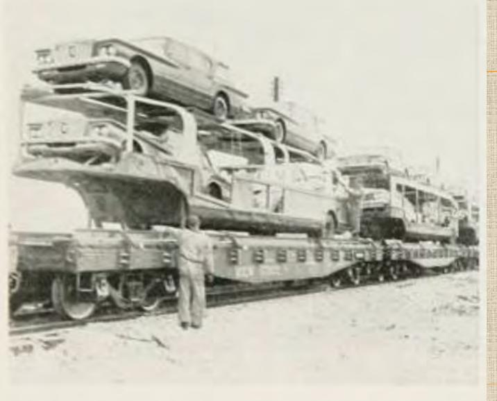
TWO FLATS with identical numbers form 90-foot underbody on Milwaukee Road for Chicago-Spokane load of 8 Chrysler Valiants and Plymouths. Carrying multideck highway trailers likely led to the elimination of the trailer in favor of the multi-deck frame directly on a car -
