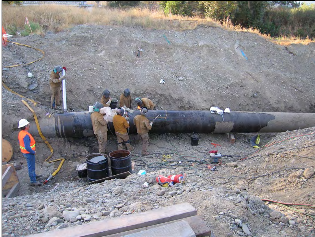
The initial cut is made.
