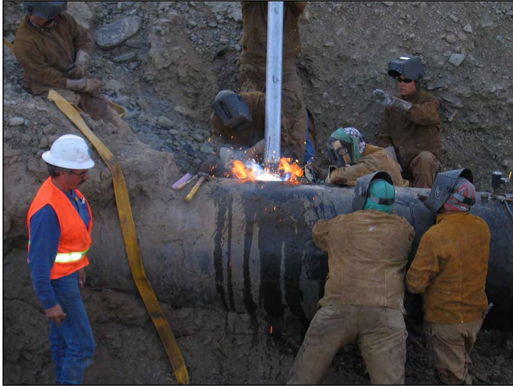
Then they weld on the control pipe.
